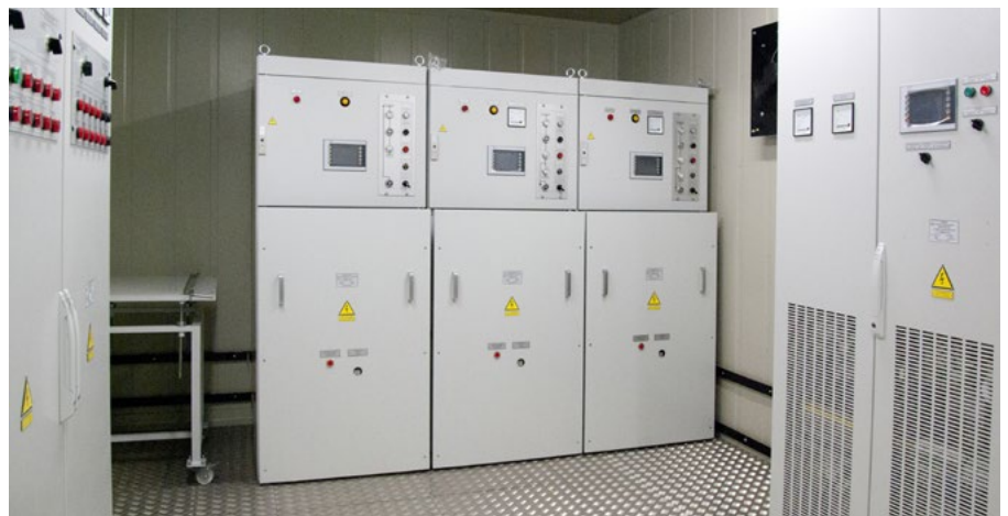
▲ Switchgear compartment. DC switchgear, rectifier, auxiliaries cabinet
